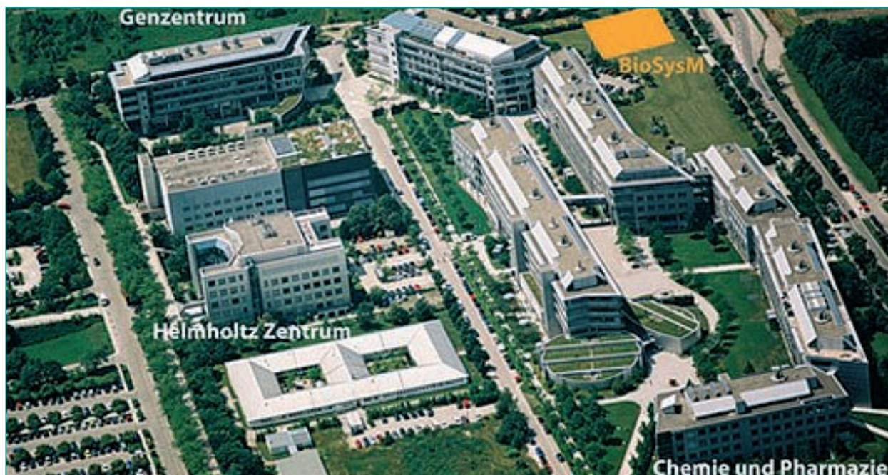
Fig. 2: The site of the planned Research Building on the campus Großhadern/Martinsried ■
